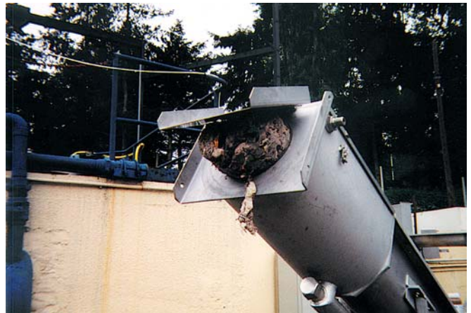
Compacted refuses outlet.
